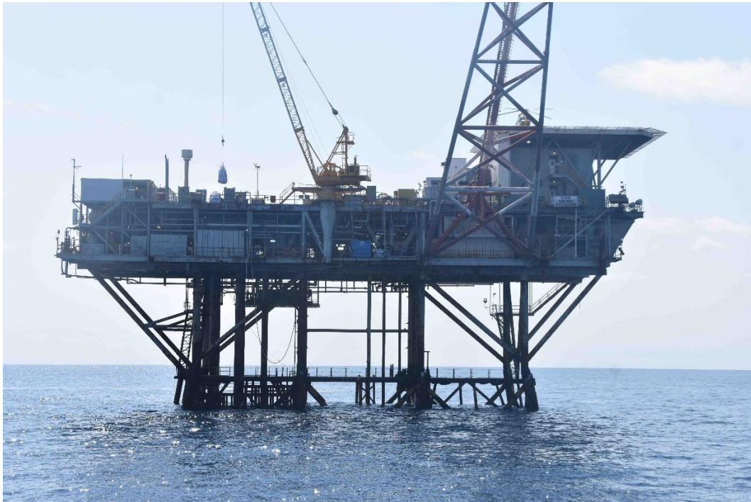
Figure 2. South Marsh Island Platform 99A. Date unknown. Source: Cox Operating.
